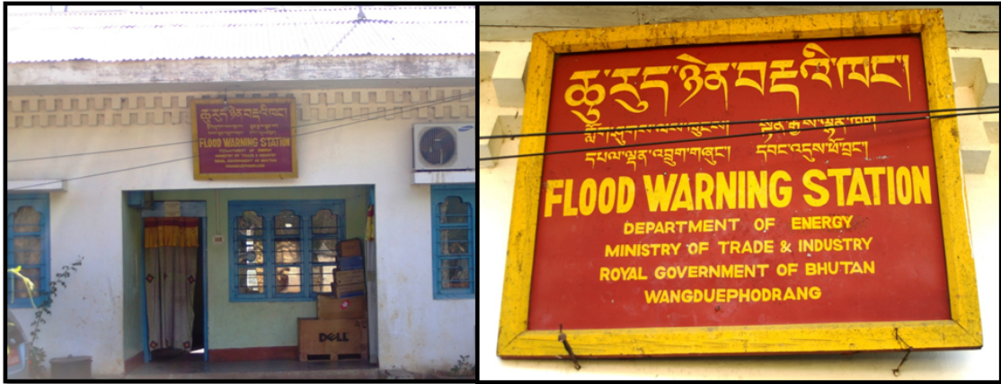
Figure 1. Flood Warning Control Station in Wangduephodrang.
