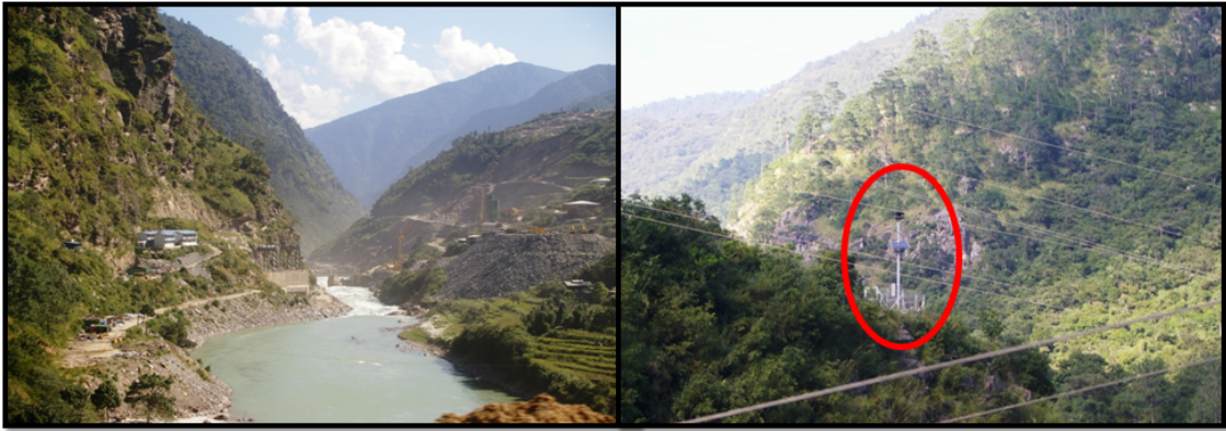
Figure 10. Location of the Punatsangchhu Dam and siren site.
